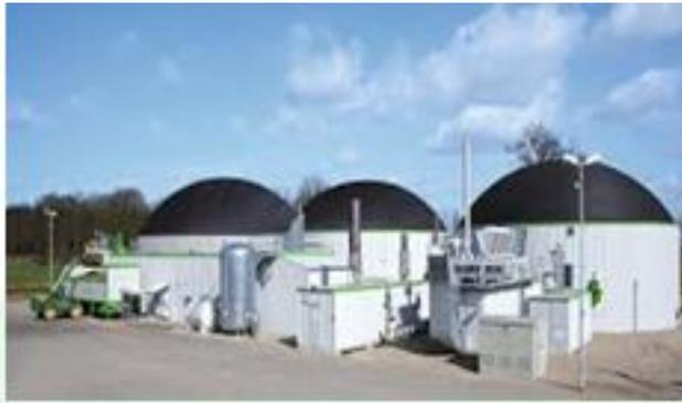
degradation producing methane-rich biogas and the sludge. The biogas production ranges from 50-150m<sup>3</sup>/ton of wastes, depending upon the composition of waste. The biogas can be utilised either for cooking/heating applications, or through dual fuel or gas engines or gas / steam turbines for generating motive power or electricity. The sludge from anaerobic digestion, after stabilisation, can be used as a soil
